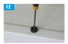
Find the centre point for the post block(s) and pilot drill a 3mm hole. Fix block in position with a No8 x 25mm pan head screws.
