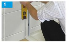
Place compensators against the wall ensuring that they rest on the flat area of the tray or floor at the position shown. Mark off fixing holes on the wall when level.
