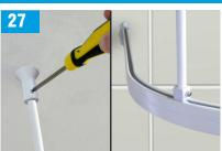
Secure drop rod into ceiling rose and rail connector into the top side of the curtain rail by tightening their respective fastening screws.
