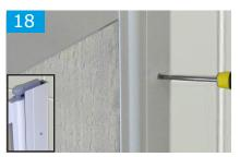
On completion of building the unit, fix the locking screws and caps into both sides of the compensators. Pilot drill two holes to the inside & two holes to the outside of the compensators & secure in position with the supplied pan head screws and grey cover caps, see inset.
