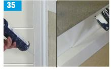
**IMPORTANT:** Seal all joints between compensators, walls, panels and shower tray or floor, on the inside and outside of the shower area using silicone sealant.
