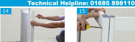
If fitting a post compensator, inline or off a return panel, place the compensator against the post and mark through the fixing slots. Find the centre of your mark and drill a 3.8mm dia hole. Fix in place with No8 x 25mm pan head self tapping screws. Offer door into post compensator as described in steps 4 to 8.
