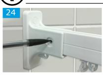
Place curtain rail into wall brackets Mark holes onto curtain rail through wall bracket on both sides and pilot drill rail with a 4.5mm diameter drill.
