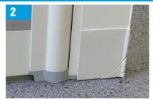
If fitting your enclosure on a wet floor, a corner block at the base of each compensator can be shaped at 10mm or 38mm radius to accept floor coving.
