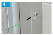
Offer door(s) / fixed panel into their respective compensator ensuring that the slots engage with the adjusting screws. Tighten adjusting screw with the supplied allen key.
