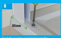
Find the centre point between the compensator. Measure 85mm and pilot drill a 3mm hole. Fix hinge locater to the tray or floor with No8 x 25mm countersunk screw.
