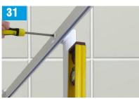
Ensuring the post is straight, pilot drill through both the curtain rail and post using a 3.0mm drill. Screw both together with a No8 x 38mm pan head screw and cap.
