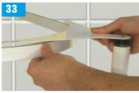
Place boomerang bracket in the top of the post, pilot drill holes in the rails top channel and fix to the post through the brackets pre-drilled holes. **REMOVE PLASTIC DUST COVER FIRST.**
