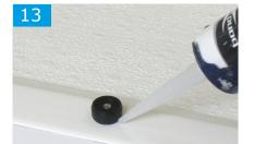
Place a small amount of silicone sealant around the post block(s) and re-fit panel assemblies in position. Fully tighten compensator adjusting screws to secure in position, as shown in Step 9.
