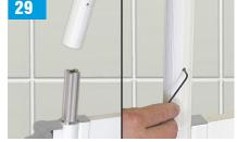
WHERE VERTICAL SUPPORT POLE IS PRESENT: With the curtain rail in position, guide the post extension over the post spigot and secure in position with the supplied grubscrew.
