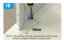
Mark hole through the panel fixing bracket onto the tray or floor & bottom rail (when door and / or fixed panel are inline). Pilot drill and fix bracket in place using self tapping screws and grey caps provided.
